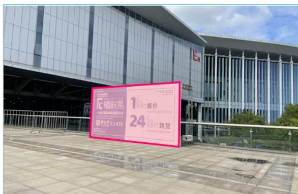
B30 Billboard – East Square (mezzanine floor)
