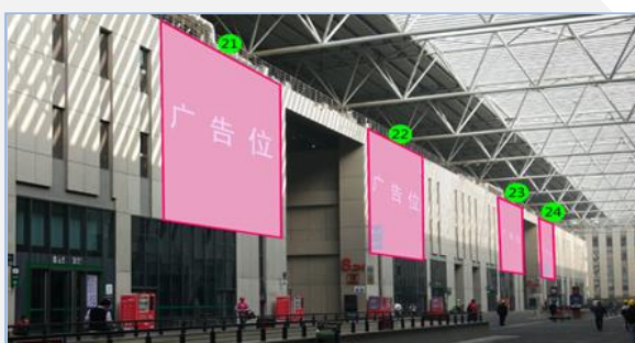
C50 Wall advertisement – Hall external on second floor
